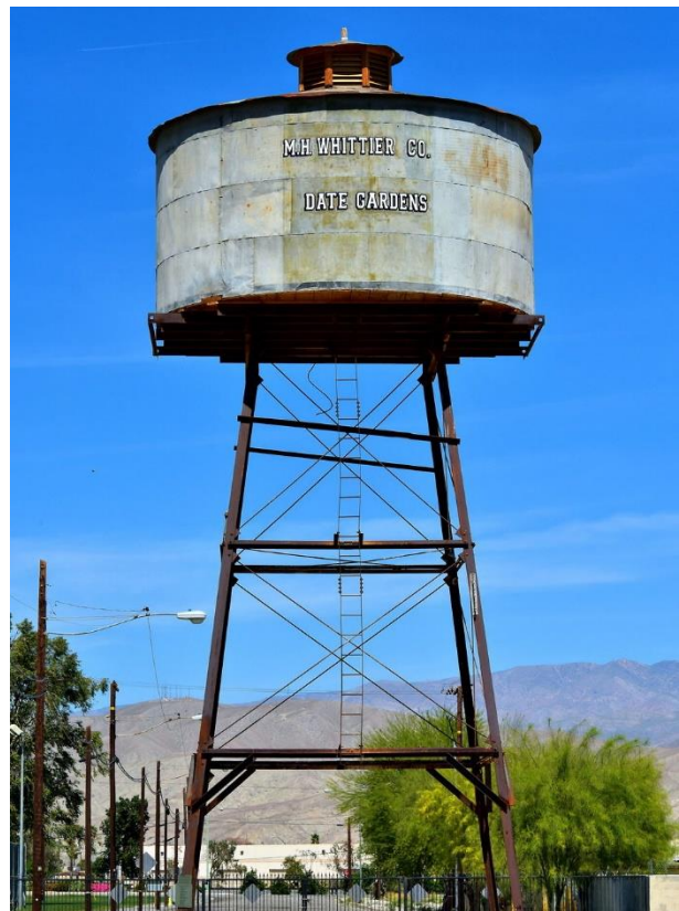
Indio’s water tower at the Date Museum
