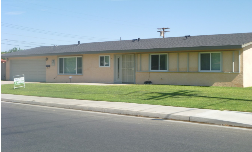
Photo of Property After Renovation.
