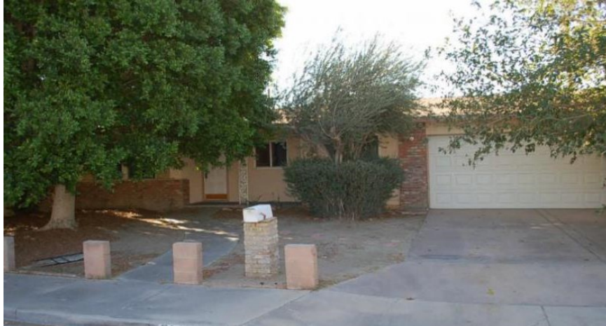
Photo of Property Before Renovation.
