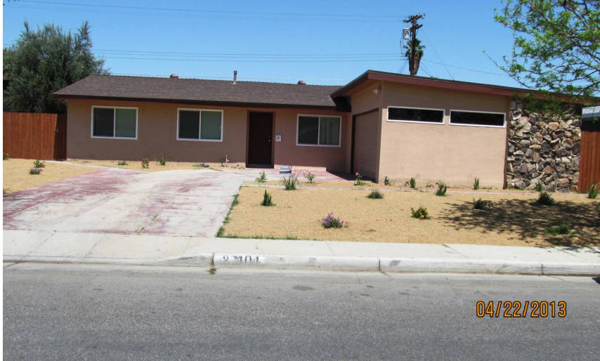
Photo of Property Before Renovation.
