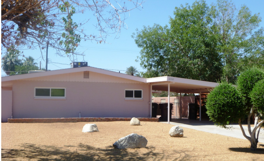
Photo of Property After Renovation.
