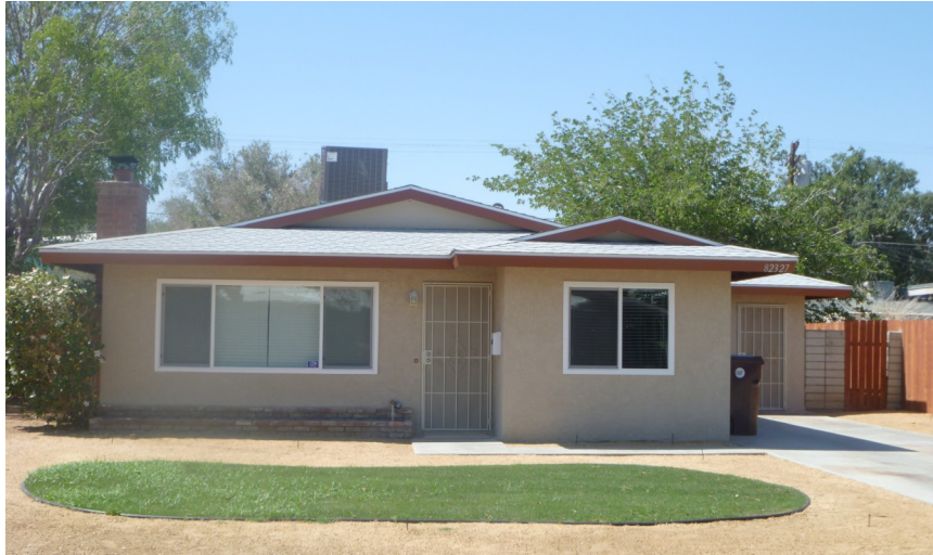
Photo of Property After Renovation.
