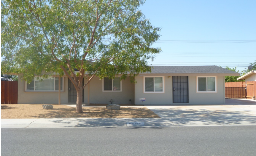
Photo of Property After Renovation.
