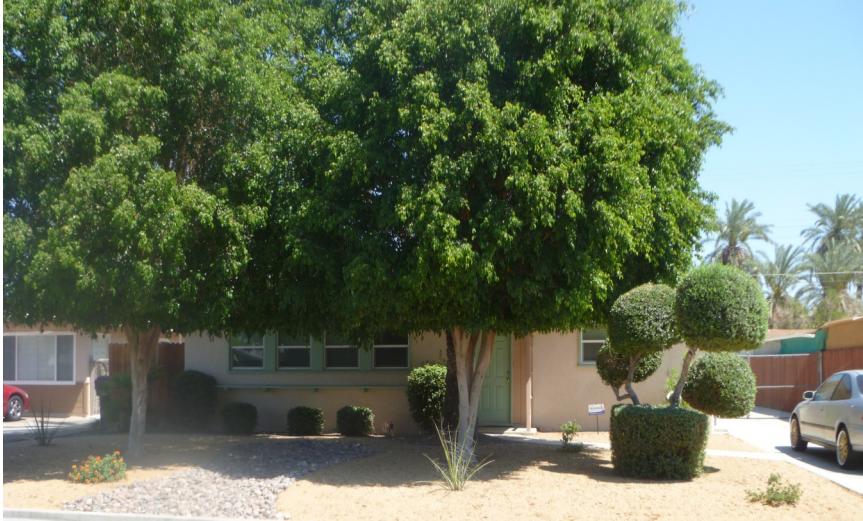
Photo of Property After Renovation.
