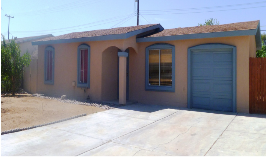
Photo of Property After Renovation.
