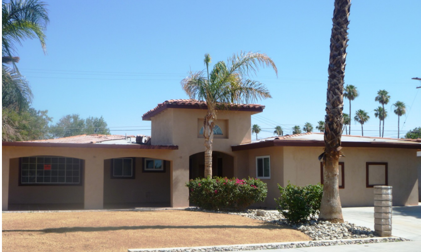
Photo of Property After Renovation.
