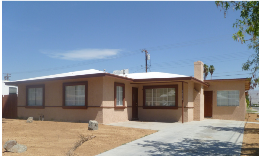
Photo of Property After Renovation.
