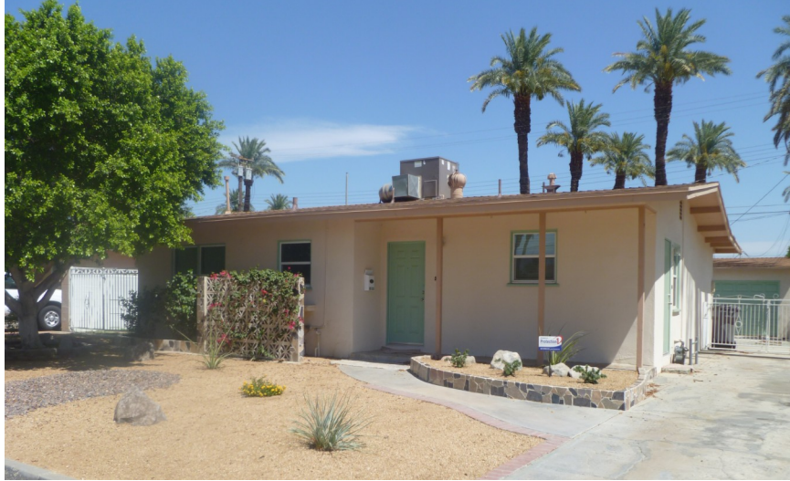
Photo of Property After Renovation.
