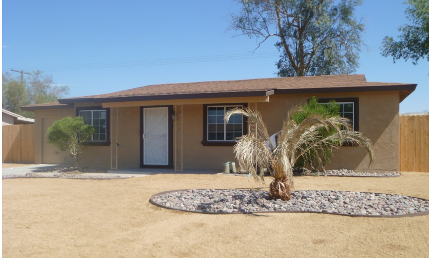
Photo of Property After Renovation.
