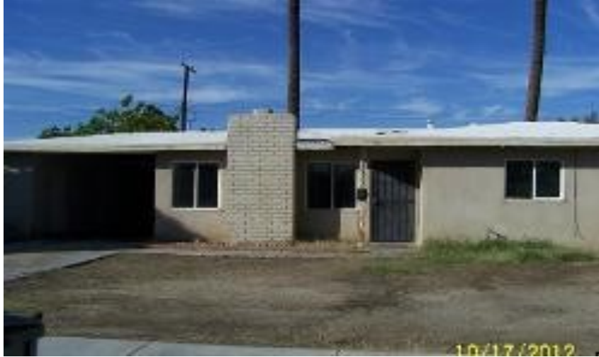
Photo of Property Before Renovation.
