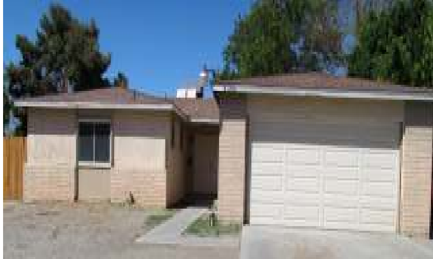
Photo of Property Before Renovation.
