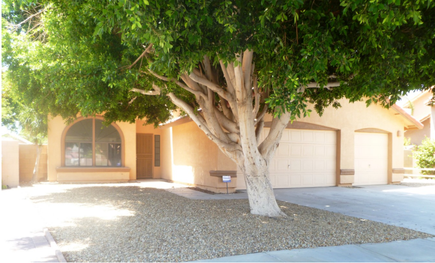
Photo of Property After Renovation.
