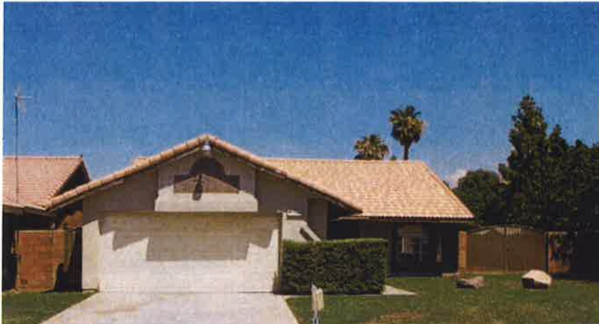
Photo of Property Before Renovation.
