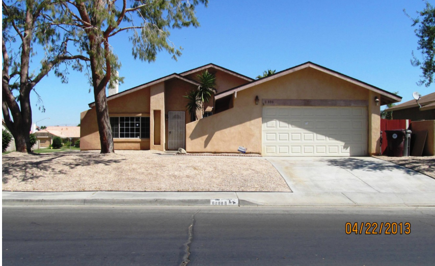
Photo of Property Before Renovation.
