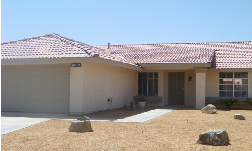
Photo of Property After Renovation.
