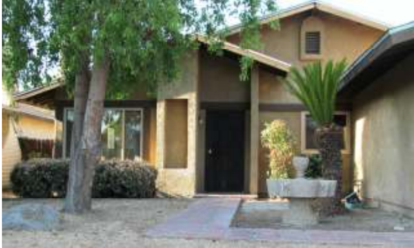
Photo of Property Before Renovation.
