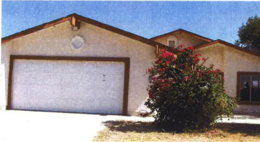
Photo of Property Before Renovation.
