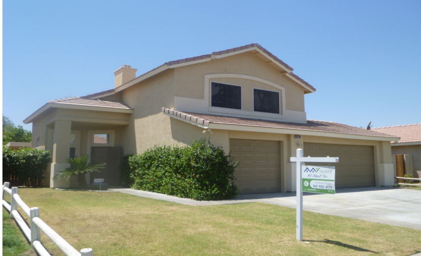
Photo of Property After Renovation.
