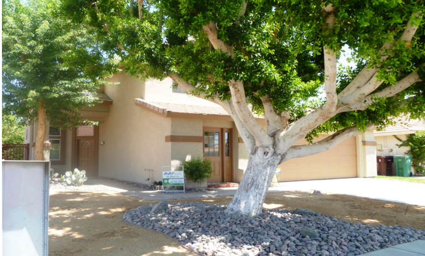
Photo of Property After Renovation.
