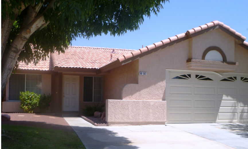
Photo of Property After Renovation.
