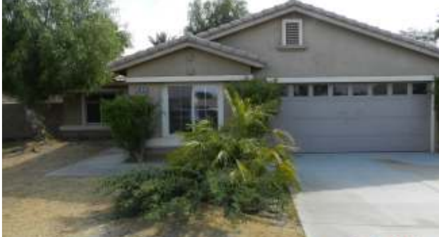
Photo of Property Before Renovation.
