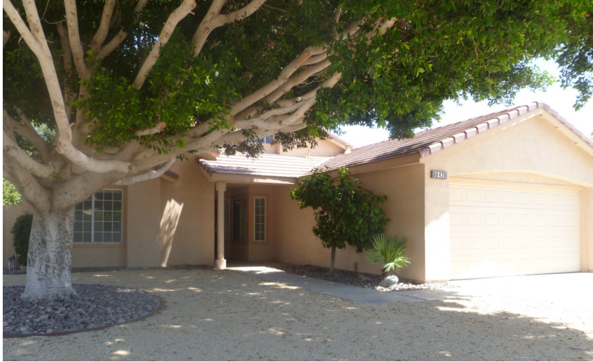
Photo of Property After Renovation.
