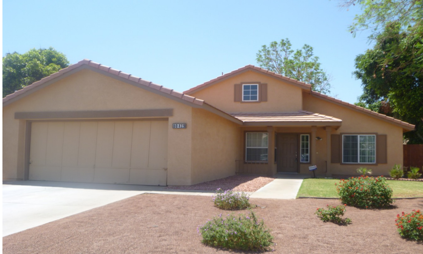
Photo of Property After Renovation.
