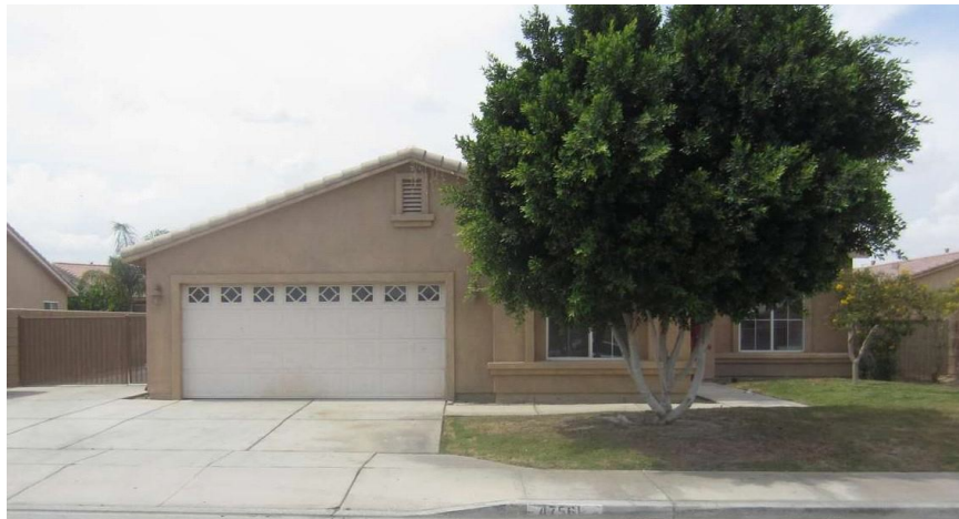
Photo of Property Before Renovation.
