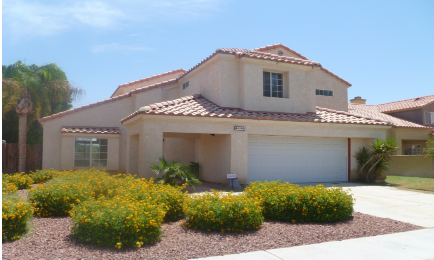
Photo of Property After Renovation.
