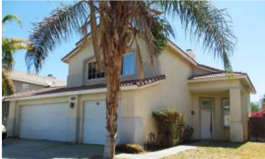
Photo of Property Before Renovation.
