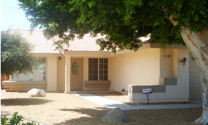
Photo of Property After Renovation.
