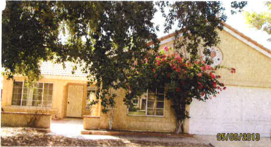
Photo of Property Before Renovation.
