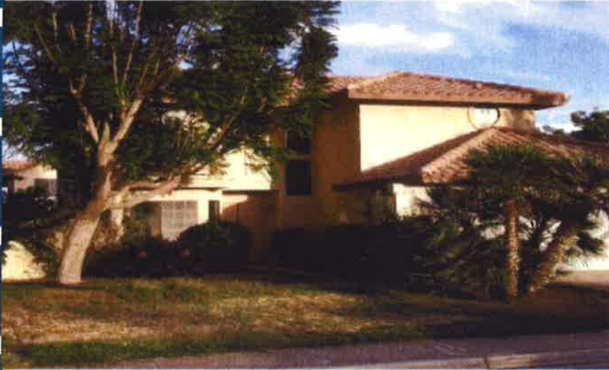
Photo of Property Before Renovation.
