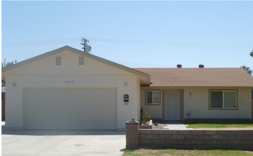
Photo of Property After Renovation.
