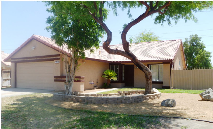
Photo of Property After Renovation.
