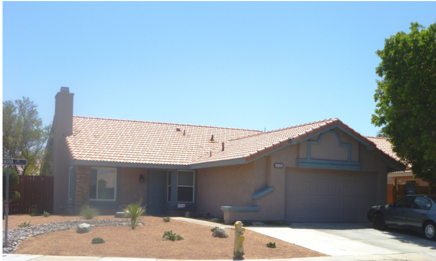
Photo of Property After Renovation.
