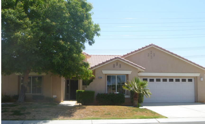
Photo of Property After Renovation.
