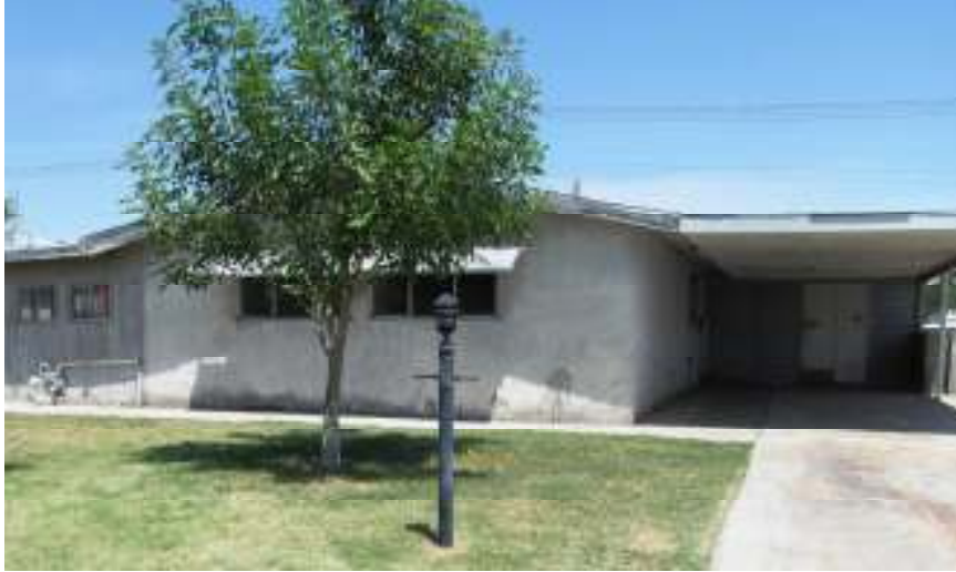
Photo of Property Before Renovation.
