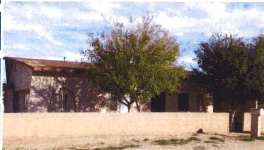
Photo of Property Before Renovation.
