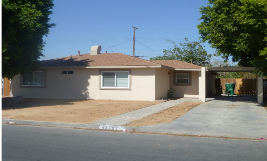
Photo of Property After Renovation.
