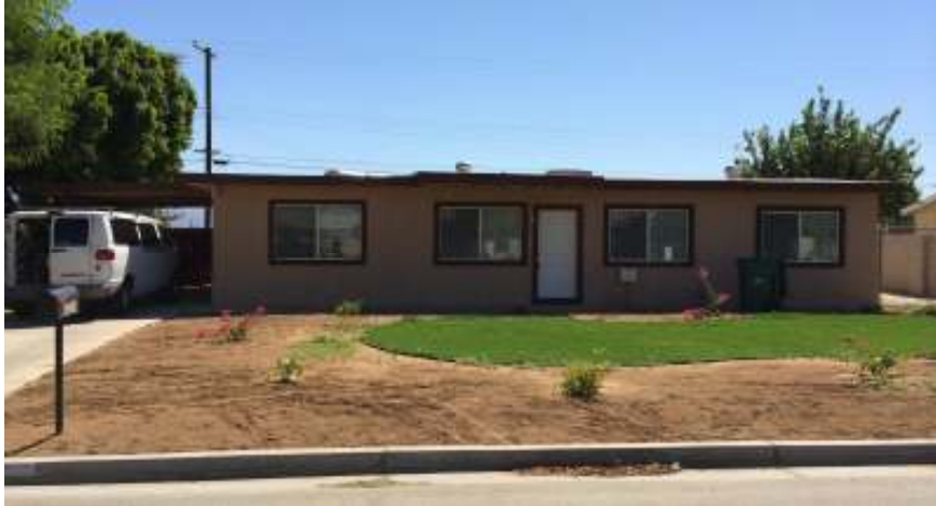
Photo of Property After Renovation.
