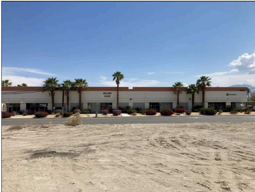
4 - View of Adj Property to the South
