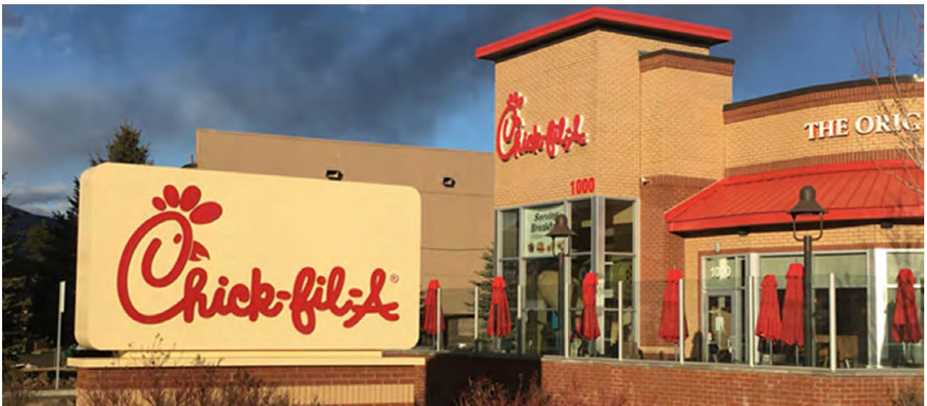
FIGURE 3.05.06-6. Example of a Freestanding Sign Incorporating the Architectural Details of the Main Building
