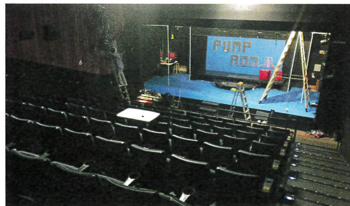
Set construction is underway in Old Towne Playhouse, the IPAC venue where Desert Theatreworks presents its plays. (By Steve Talbot)
