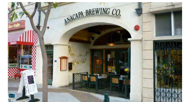
Recessed shopfronts can provide opportunities for active uses like outdoor dining, without interrupting the streetwall.
