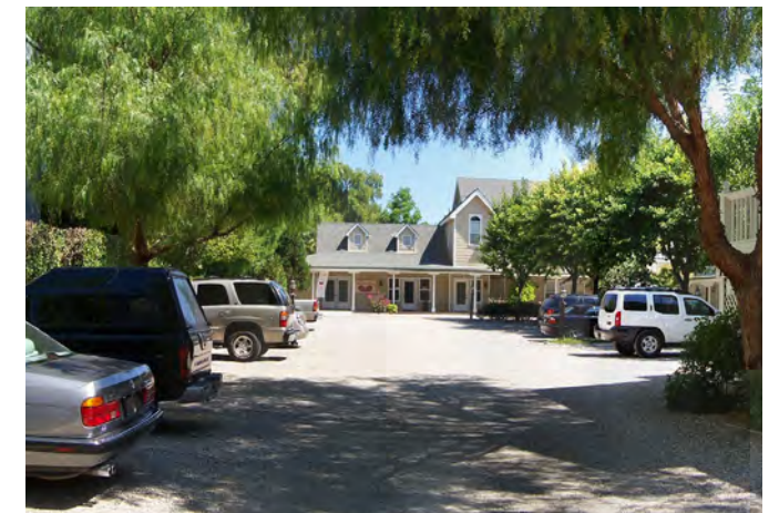
A parking lot paved with gravel allows water to infiltrate, reducing runoff.
