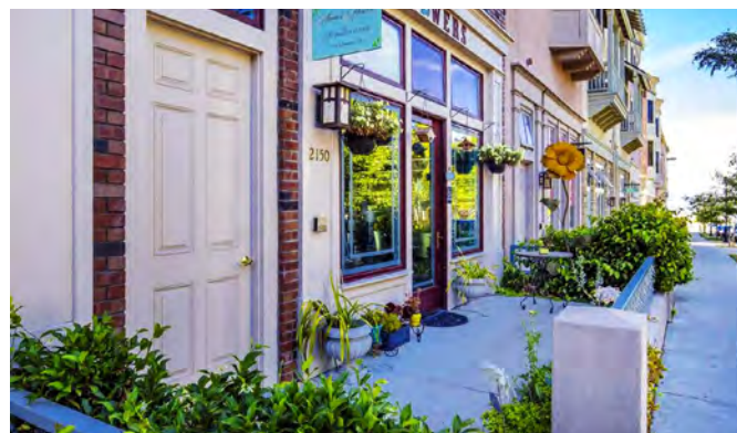
An example of the form (not style) intended for the Retail-Ready Overlay. Where the market is not ready for retail, ground floors may be designed for residential or office use in the meantime.
